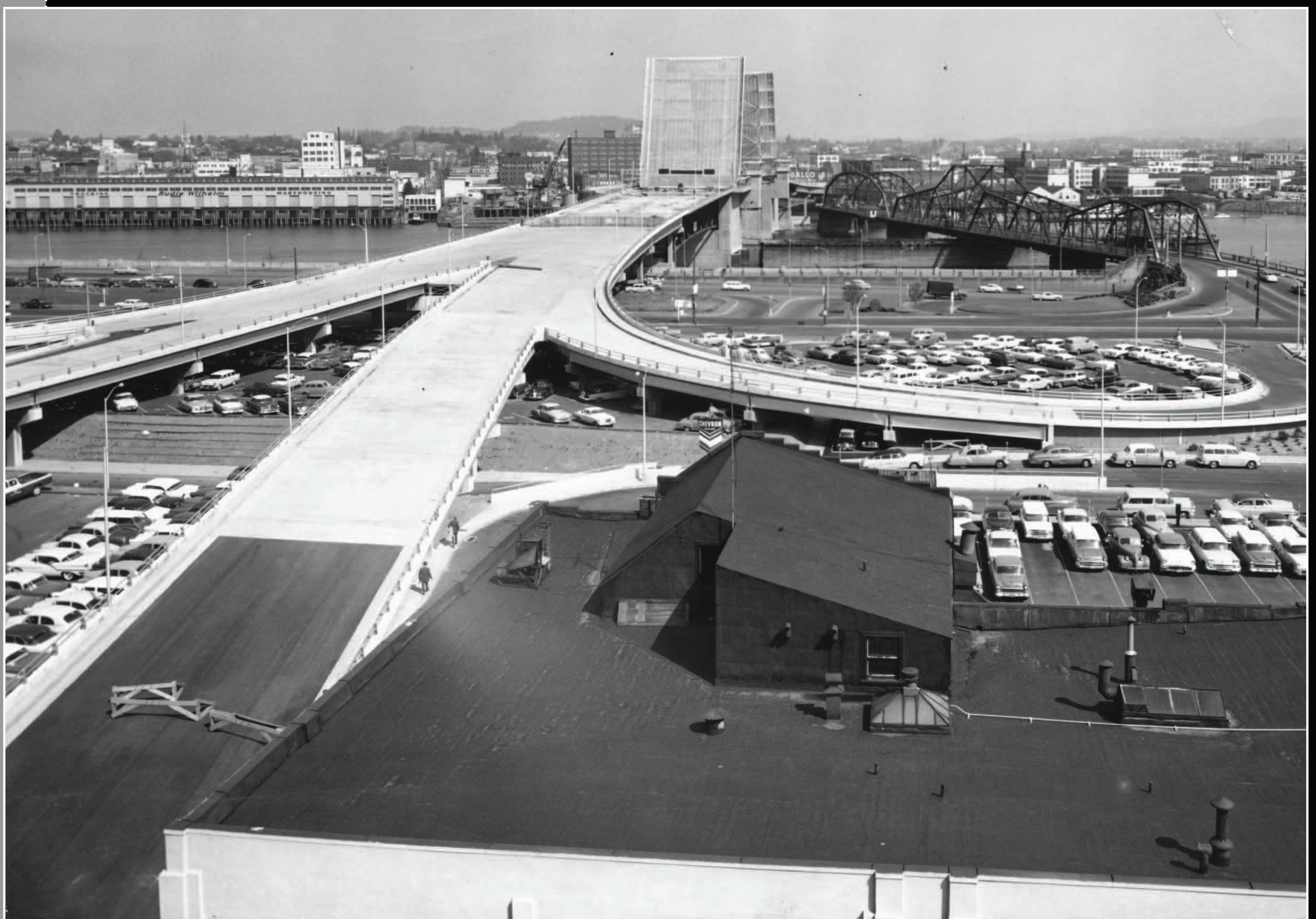
CONSTRUCTION OF THE NEW MORRISON BRIDGE, 1958
